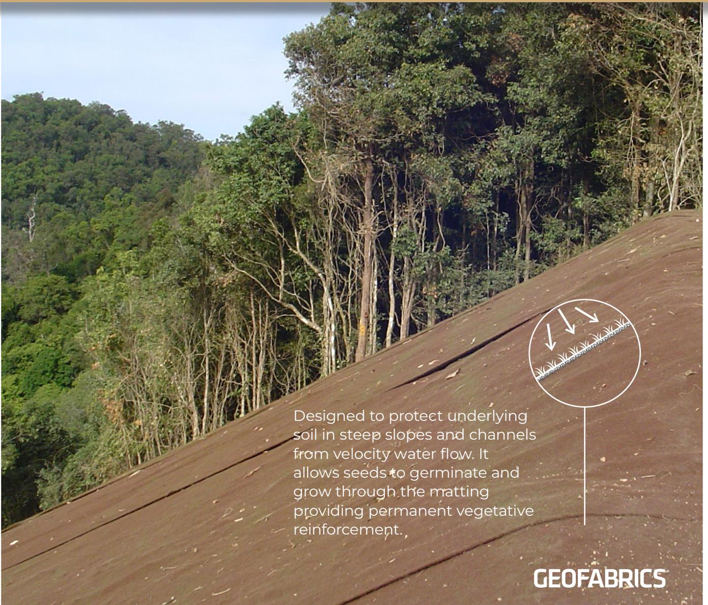
Designed to protect underlying soil in steep slopes and channels from velocity water flow. It allows seeds to germinate and grow through the matting providing permanent vegetative reinforcement.
