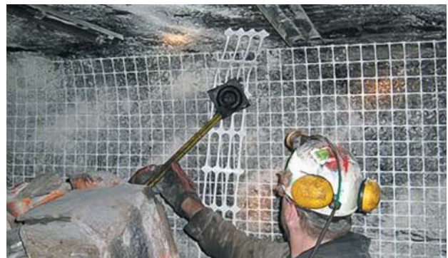
Tensar UX Rib Straps, when combined with Tensar Mining Grid and Minex Rock Mesh, enhances the strength of the underlying mesh.
