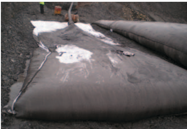
Tensar® Geotextile Tubes can contain even fine grained, highly organic materials.
