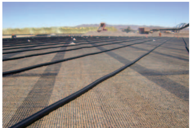
Tensar Geogrids provide additional bearing capacity over leachate collection systems to support heavy equipment loads.
