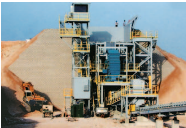
Tensar Grade Separation Solutions can be built using a wide range of backfill materials and a variety of facing types.
