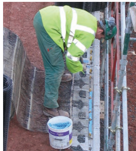
A feature common to all TensorTech™ Wall Systems is the high efficiency connection between geogrid and facing unit, which is quick and easy to install.
