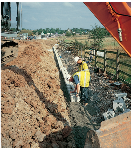
TensorTech™ TW3 concrete blocks are dry laid, without mortar.
