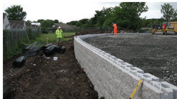
TensarTech™ TW3 facing units are simple to install and can easily accommodate tight concave or convex horizontal curves.
