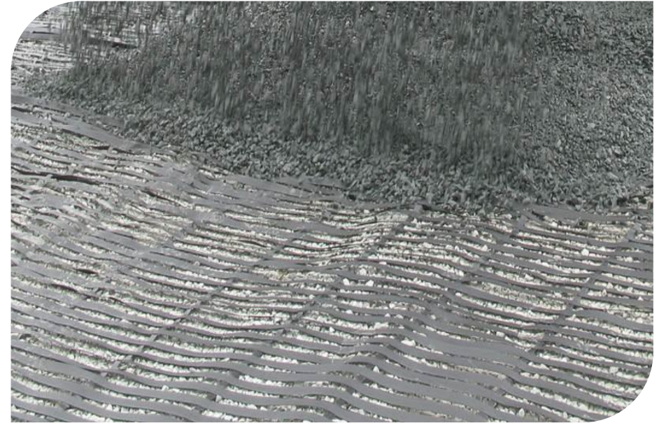
Installation of ParaGrid
