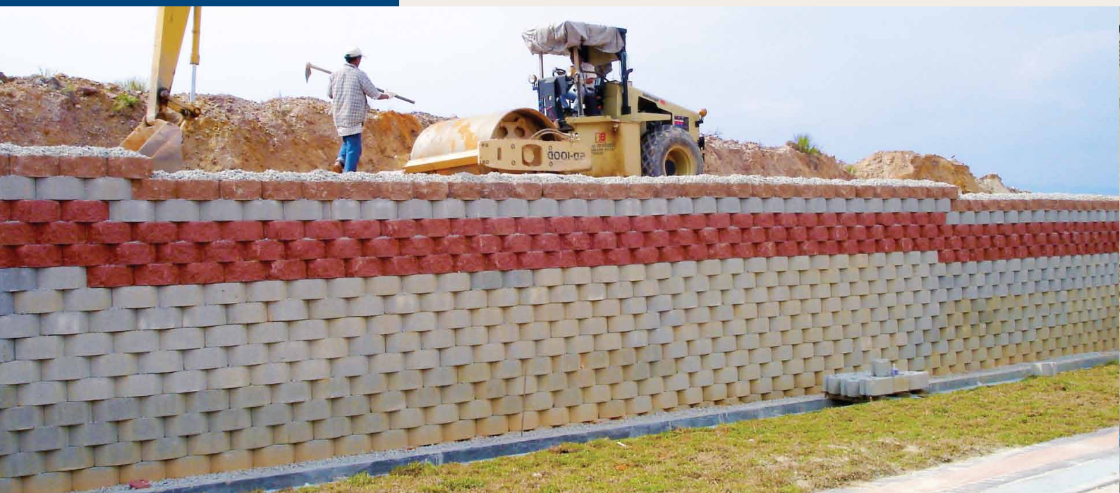
Reinforcing with Miragrid® GX geogrids.
