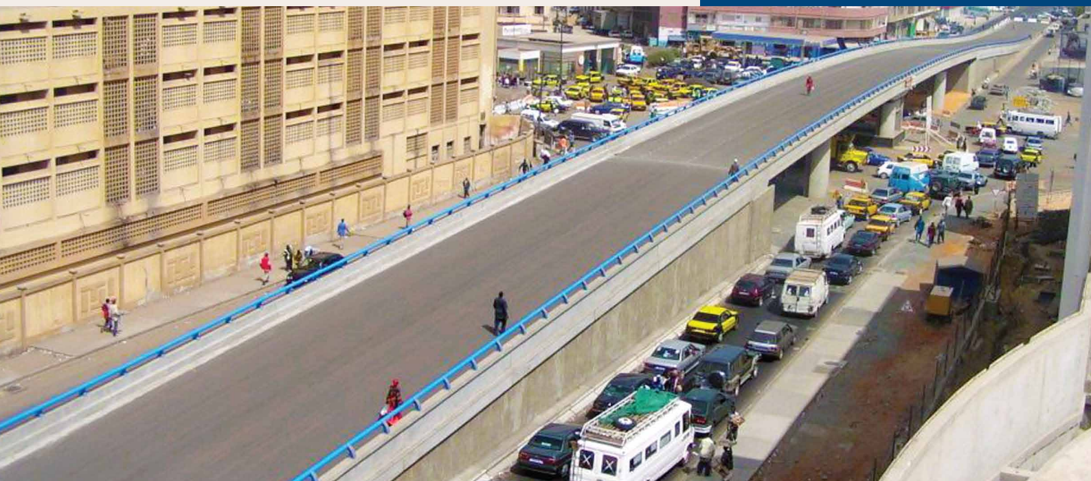
Reinforced soil wall during construction.
