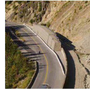
1 Rockfall and Landslide Embankments
