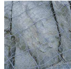
3 Mesh Systems - Secured Drapery / Surface Stabilisation
