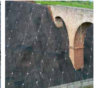
6 Soil Nailing and Surface Protection
