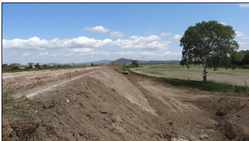
Fig. 7 – Mattresses foundation levelling
