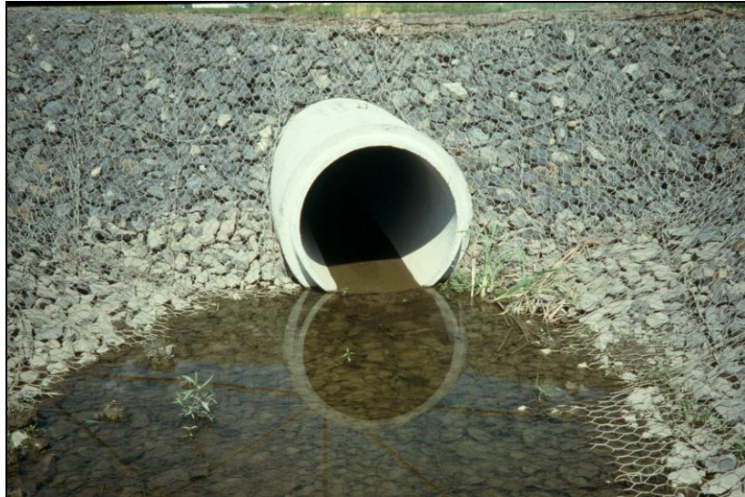
Fig. 21 - Pipe crossing through a mattress unit
