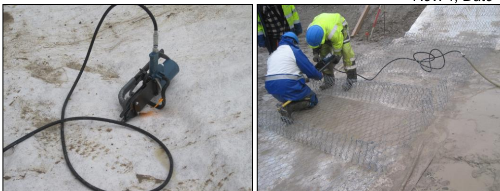
Fig. 6 – Use of the pneumatic lacing gun
