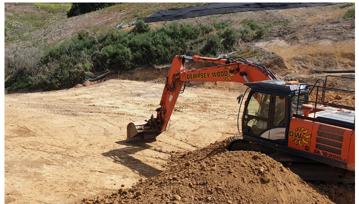
Preparation for next Paragrid layer
