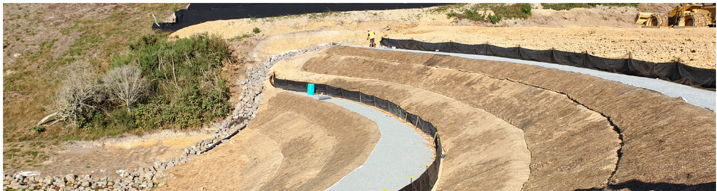
Completed structure using Paragrid and Miragrid products
