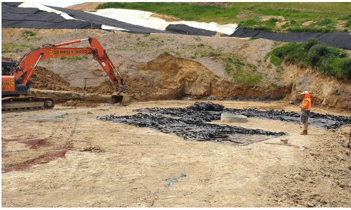
Preparation for laying of Paragrid
