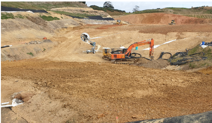
Backfill of first two layers of Paragrid
