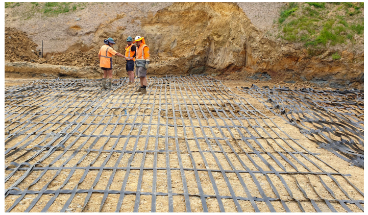
Laying of Paragrid with correct overlaps required
