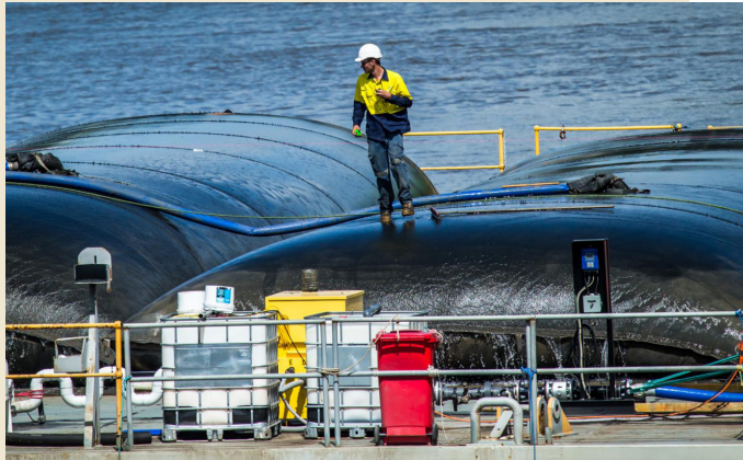
Geotube® units while dewatering.
