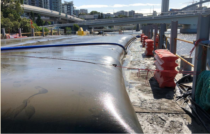
Geotube® units shown on the barge.
