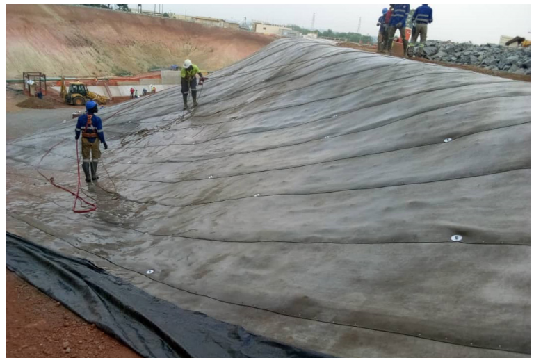
Protection of edge of last CC layer before hydration
