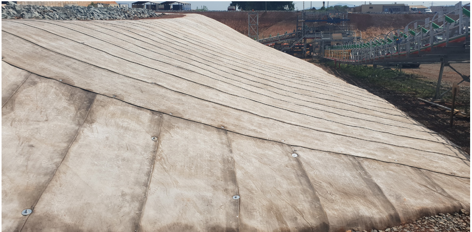
Slope protection installation incorporating warm climate installation guidance
