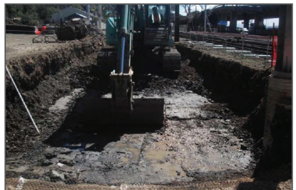
Preparation of subgrade for geotextile and first layer of geogrid
