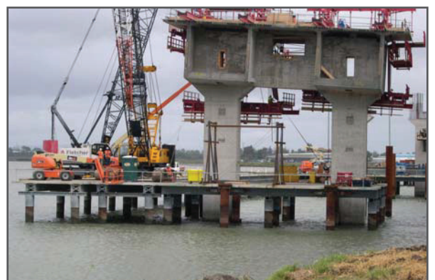
Temporary platform landing constructed
