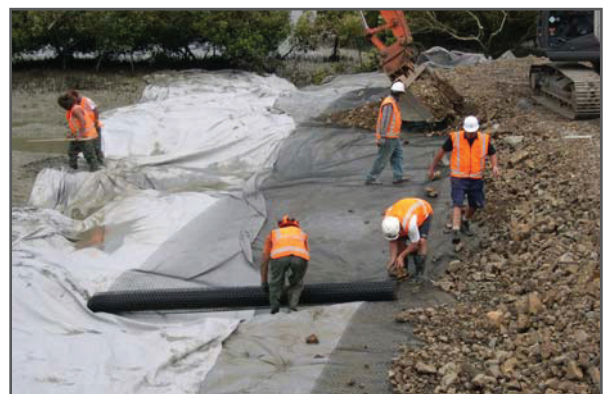
Placement of Tensar TriAx® and bidim® for landing
