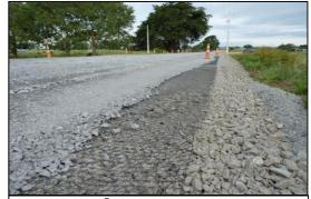
Tensar TriAx® being laid with aggregate
