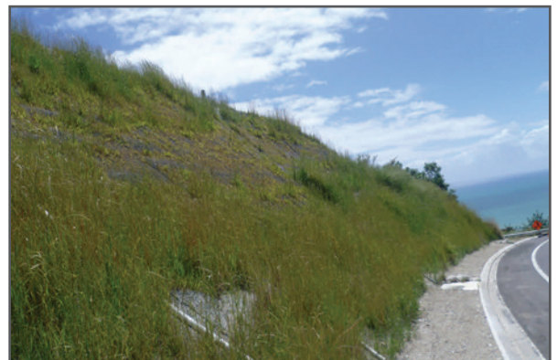
Greened up slope following construction
