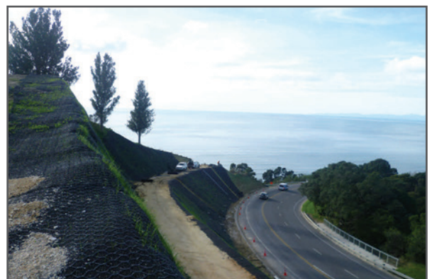
Completed MACMAT-R slope prior to hydro-seeding
