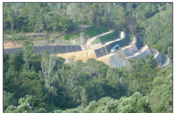
During construction on the roadside
