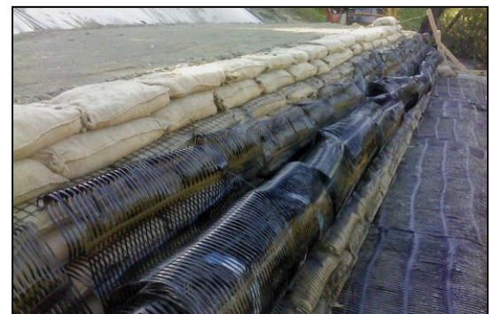
Constructed of MSE wall
