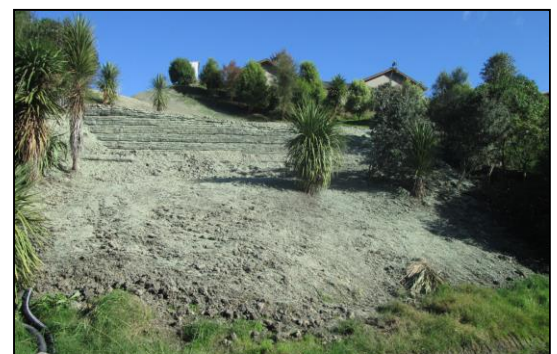
Hydro seeded wall
