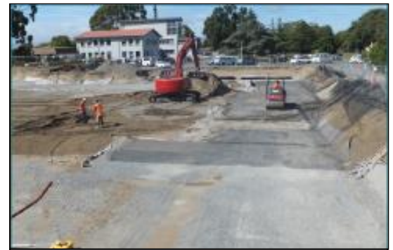
Beginning the building platform
