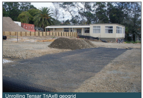
Unrolling Tensar TriAx® geogrid
