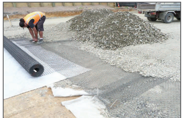
Temporarily fixing the next roll of Tensar TriAx® geogrid
