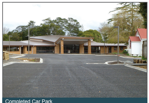
Completed Car Park
