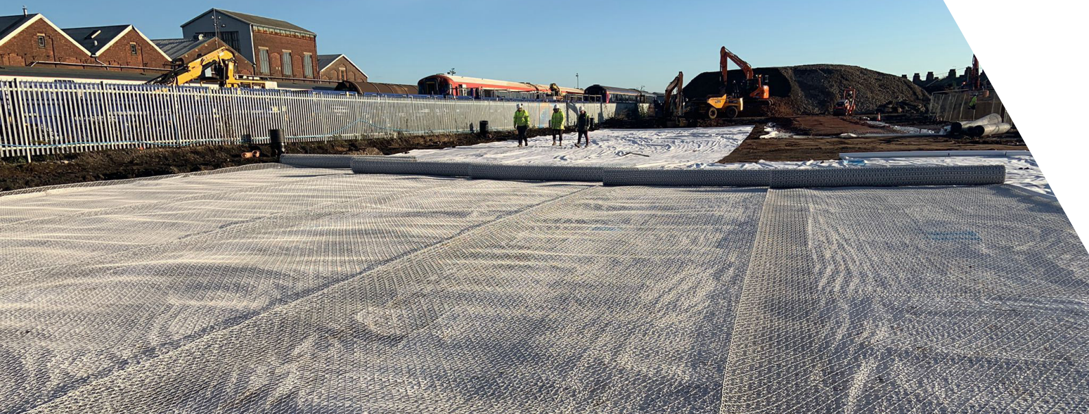
Tensor InterAx geogrid provided a two stage Mechanically Stabilised Layer (MSL)
