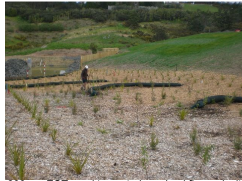
300mm ECT used to control overland flow velocity thereby removing sediment and other debris.
