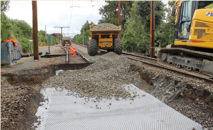
Install of Geocomposite Tracktext™ followed by Tensar TX170 geogrid.
