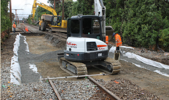
Removal of ballast, preparation of site, subsoil drain install.
