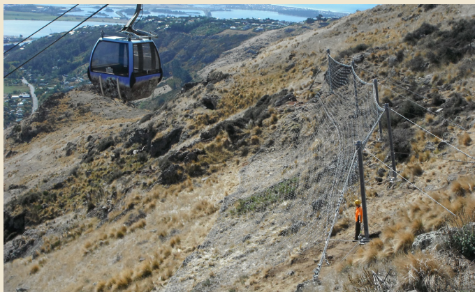
Completed attenuator fence.
