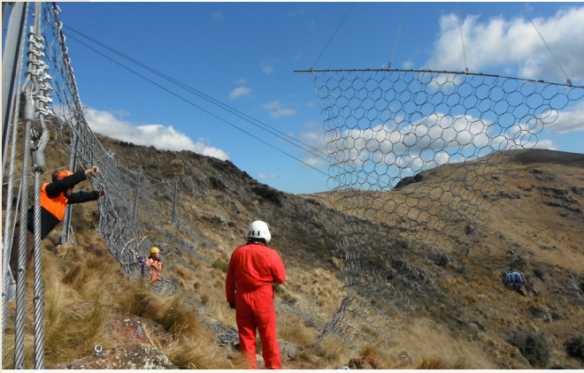
Helicopter being used to help position the drape.
