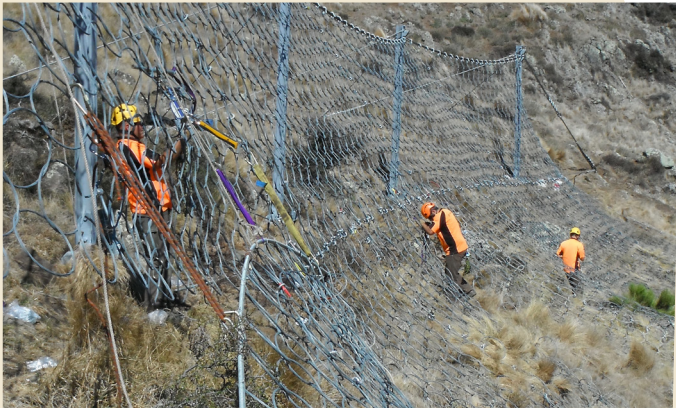
Connection of ring net panels.
