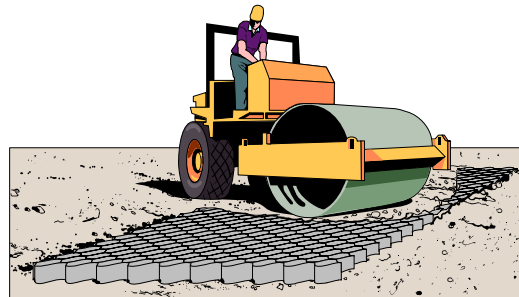
Figure 16 Infill Compaction
