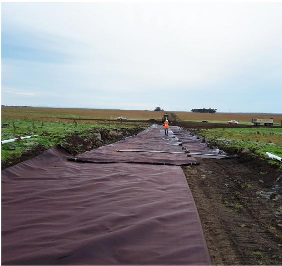
After verifying the hardstand design with different design guidelines such as Finite Element Analysis, Acciona Energía's design team accepted the use of 400mm thick Mirafi RS580i to reinforce the economical fill pavement layer over subgrade UDS of 50kPa. The unique characteristics of Mirafi RS580i allowed the contractor to place locally available economical fill material without compromising the performance of the hardstand areas.
