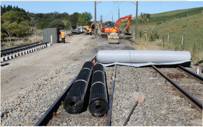
Subgrade preparation prior to product installation.
