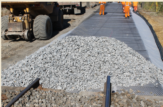
Ballast being laid on top of installed product.
