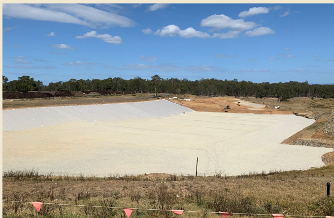
The newly constructed cell is now ready to take waste.
