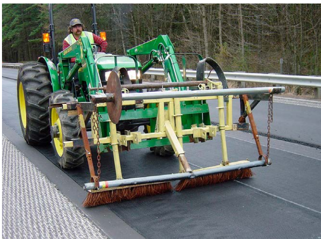
Figure 43: ADFORS GlasGrid installed only in slow lane 2006
