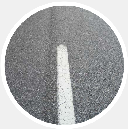
Figure 25: Section with ADFORS GlasGrid shows no cracking
