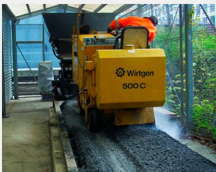
Figure 32: Milling the reinforced area
