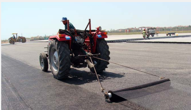
Figure 47: Installation of ADFORS GlasGrid at Atatürk Airport in 2010
