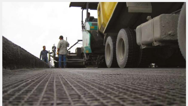
Figure 48: Installation of ADFORS GlasGrid at Atatürk Airport in 2010
