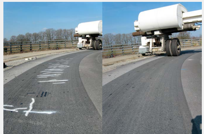
Figure 22: Reference section at the end of the test (left) Section with ADFORS GlasGrid at the end of the test (right)
