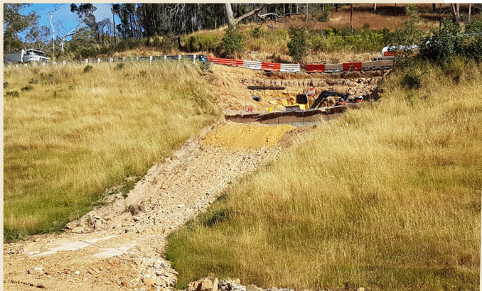
During installation of the Green Terramesh retaining system.
