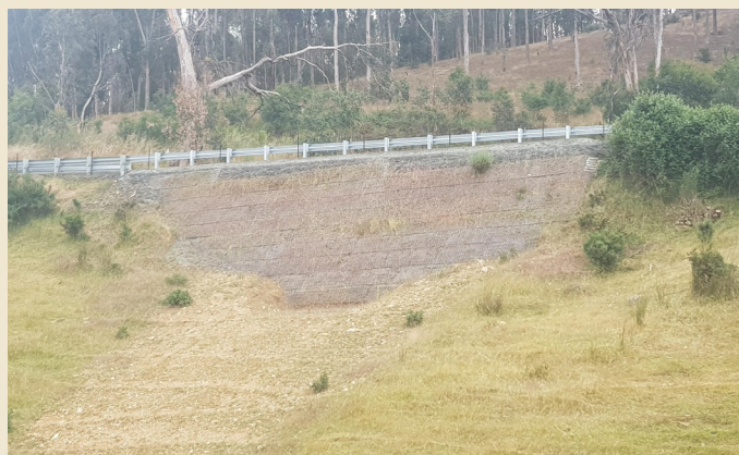
Completed Green Terramesh structure with vegetation growth.
