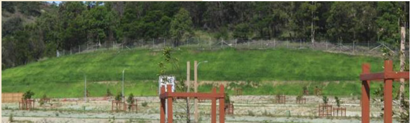
Six weeks after the MacMat R was installed - extensive vegetation establishment after hydroseeding.
