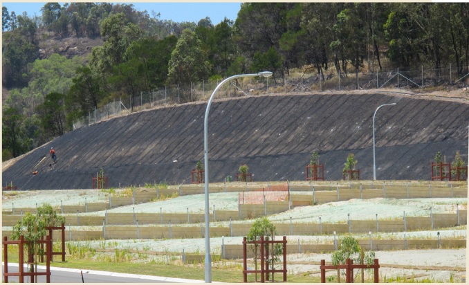
The slope after installation of MacMat® R prior to hydroseeding.
