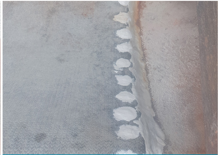
Shot-fired nails and CCX edge covered with epoxy to restore impermeability
