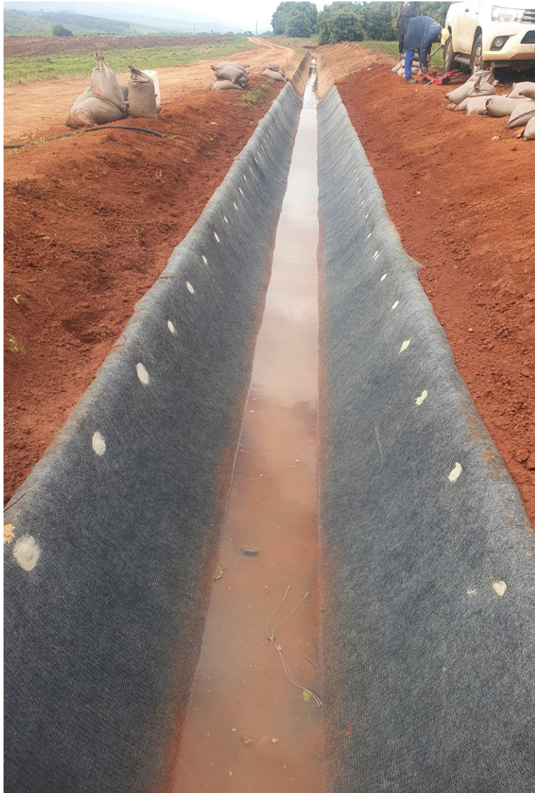
Completed installation following hydration
