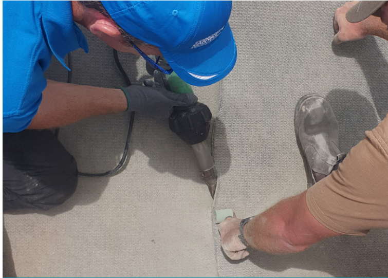
Thermal welding of CCX-M™ joint
