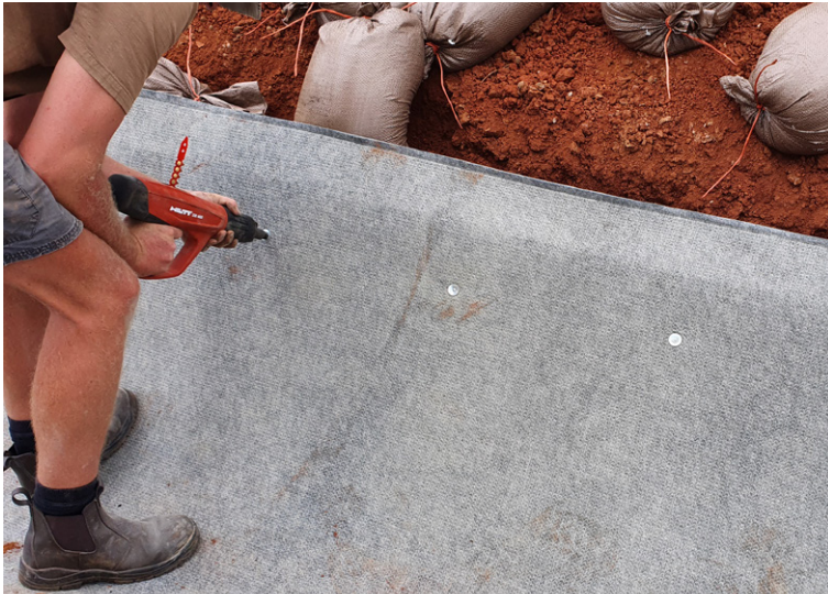
Installation of shot-fired nails
