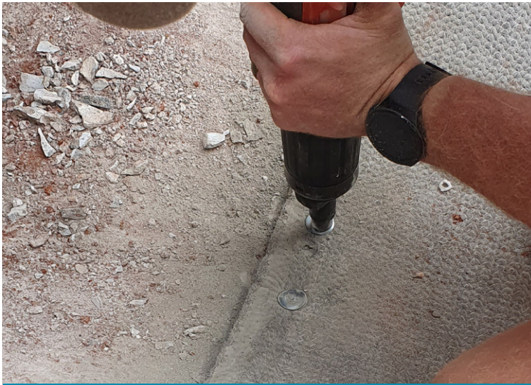
Shot-fired nails used to secure CCX-M™ edge within termination slot
