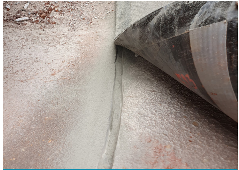
Termination slot created to secure CCX-M™ edge
