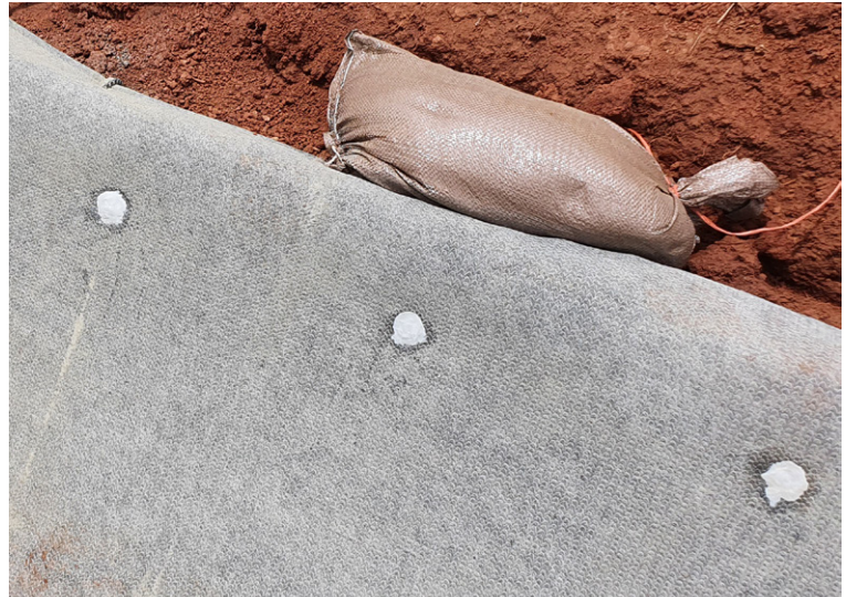
All nails were covered with epoxy
