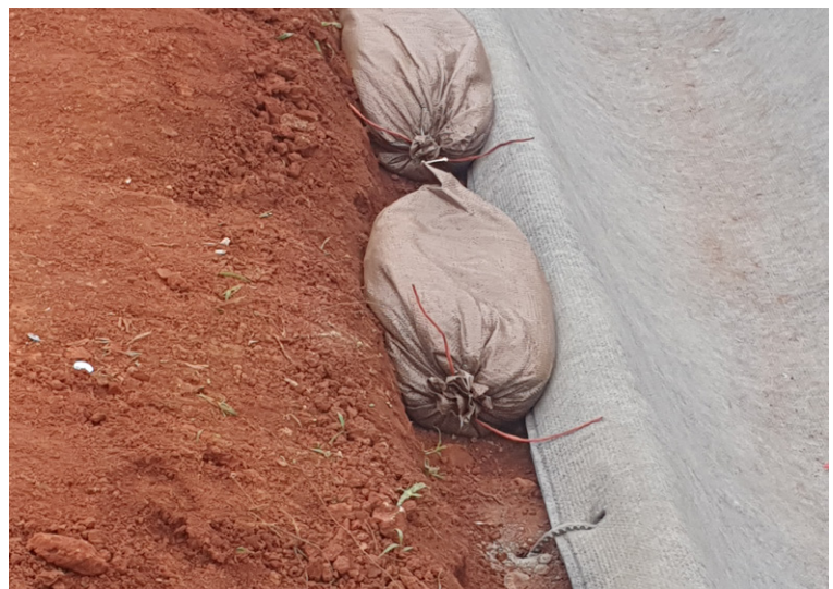
Sandbags laid over CCX-M™ edges to prevent lifting during installation
