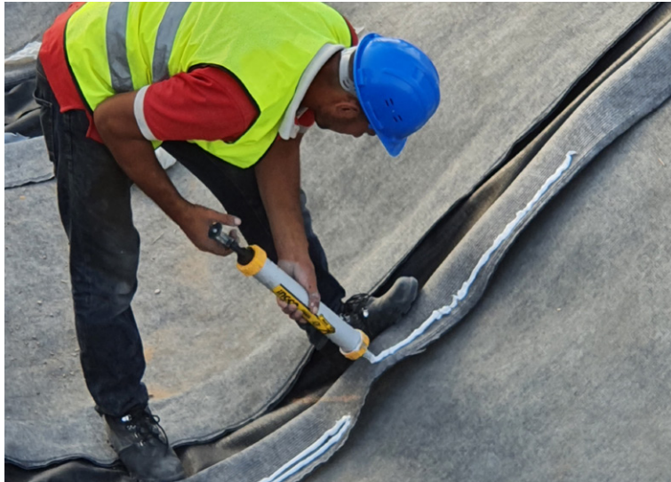
Adhesive sealant applied to overlaps
