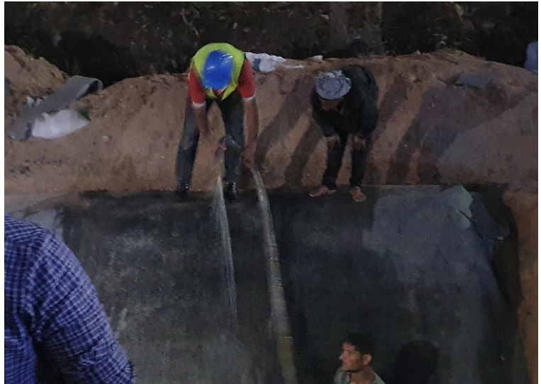
Hydration of CCX-B™ at dusk to avoid excessive evaporation
