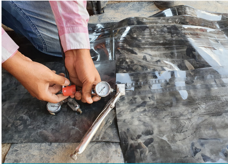
Test welds were carried out and pressure tested prior to installation
