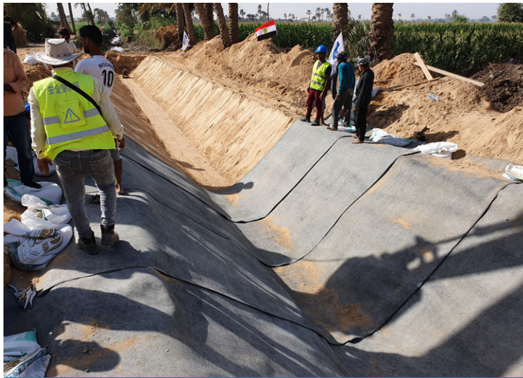
Layers of CCX-B™ overlapped by 100mm
