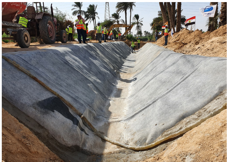
Downstream anchor trench backfilled with poured concrete
