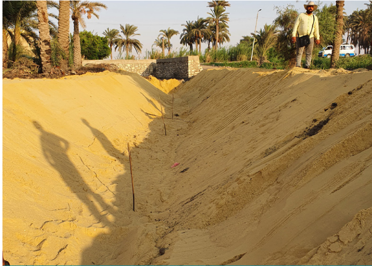
Following excavation, a sand-based gravel substrate was imported
