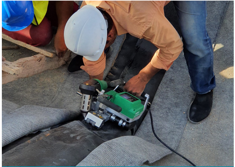
Thermally welding geomembrane backing layers
