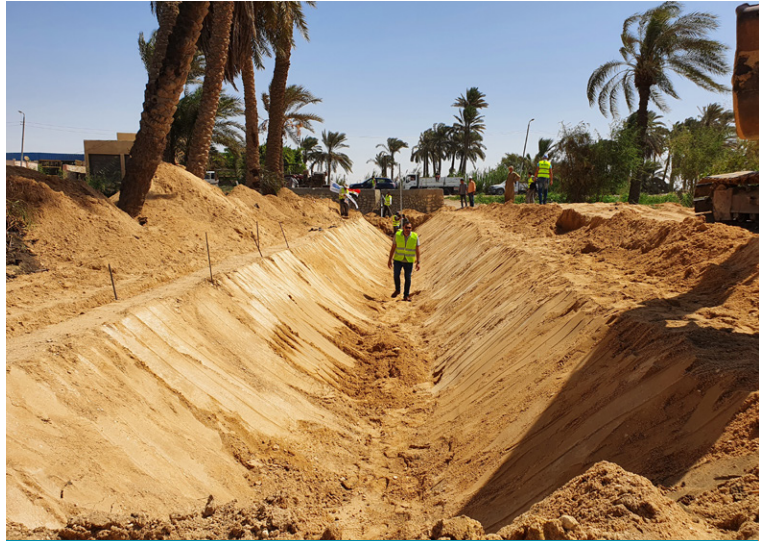
Canal profile following compaction of substrate
