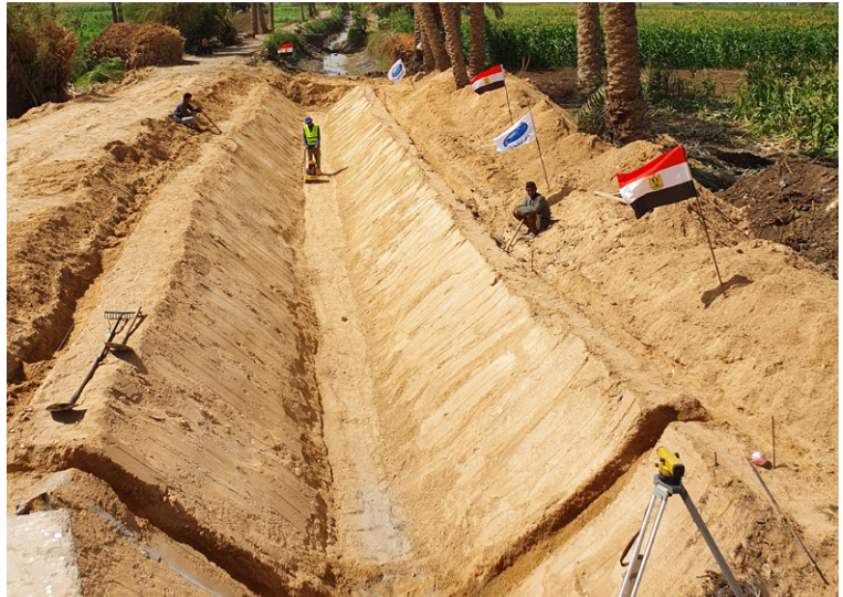
Anchor trenches created on canal shoulders and 50m termination point
