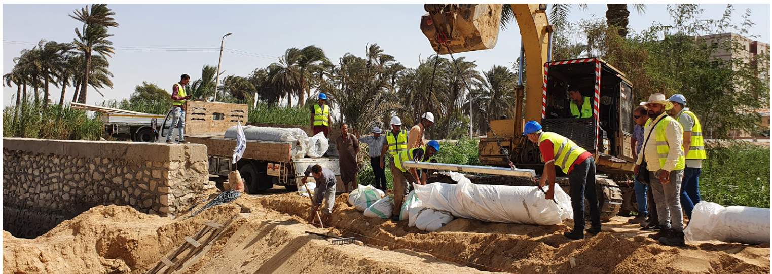
CCX-B™ rolls positioned along the canal shoulders for easier deployment
