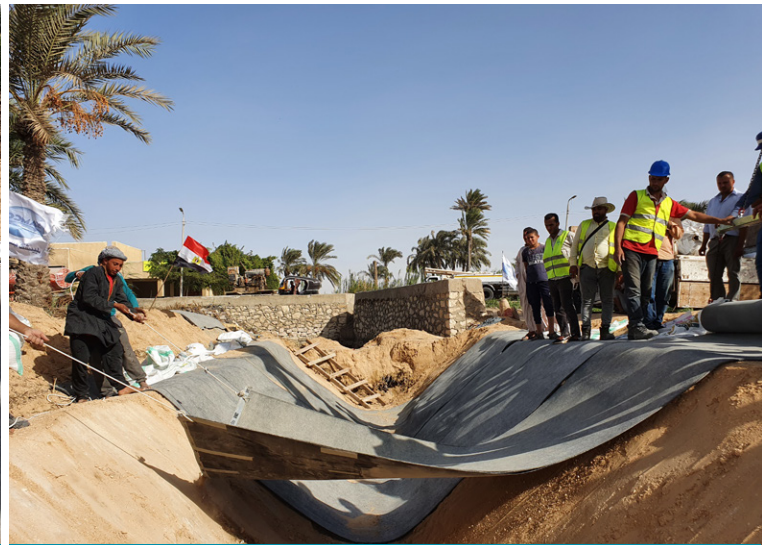
Lengths of CCX-B™ were manually pulled across the canal and positioned
