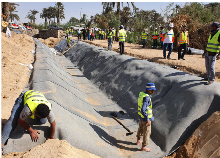
Tucking downstream edge into anchor trench
