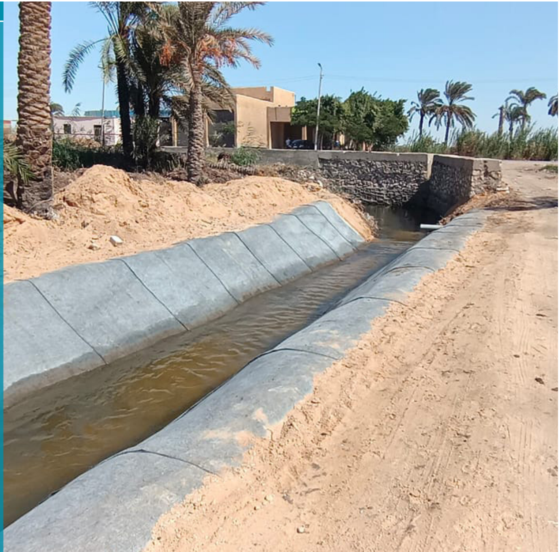
Completed CCX-B™ trial installation in Egypt
