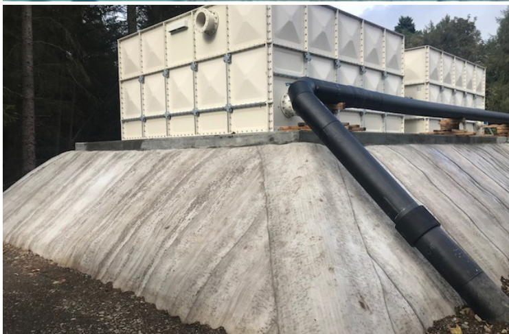
New Reinforced Soil Slope designed with CC armoured facing
