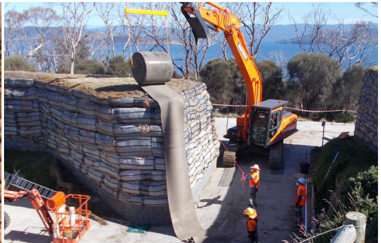
Protection of Mechanically Stabilised Earth wall to prevent animal damage
