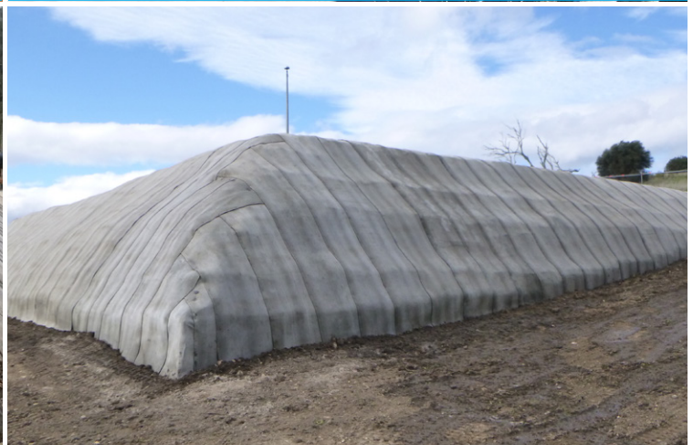
Protection of reinforced soil slope to prevent vandalism
