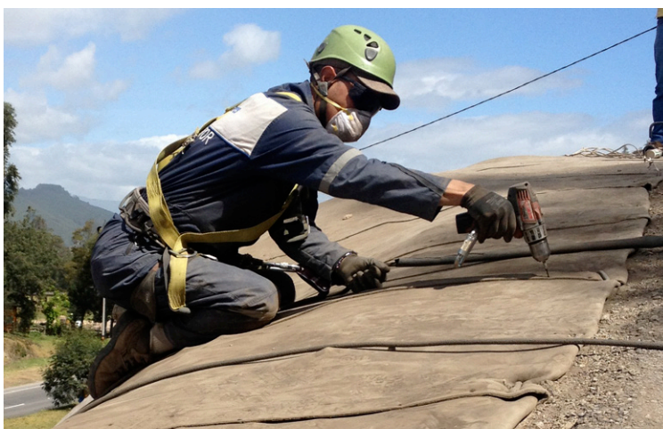
Jointing adjacent layers of CC using stainless steel screws
