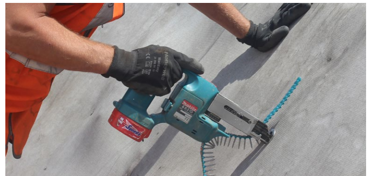
Figure 5.4 CC joint fixed using an autofed screwdriver
