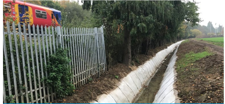
Uniform surface achieved after jet washing surface
