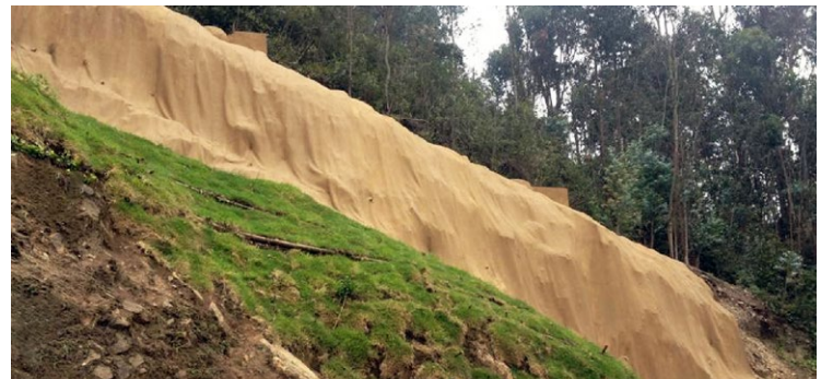
Applied coating to change aesthetic
