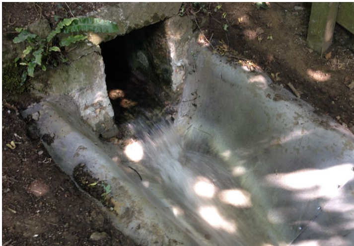
Figure 8.5 Mortar used to seal to existing infrastructure
