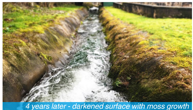
Completed CC lined channel
