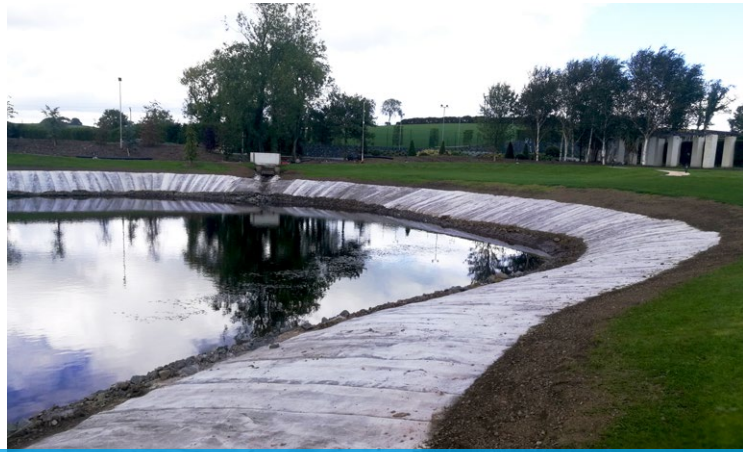
Figure 3.3 CC bank protection on a raked soil substrate (images taken before and after install)
