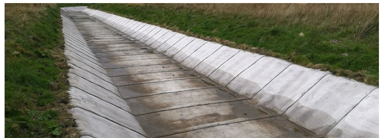
Figure 3.8 After the installation of channel remediation
