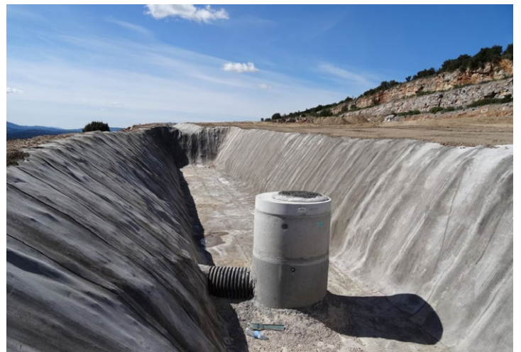
Figure 8.8 CC installed around existing infrastructure
