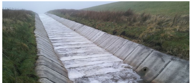
Figure 3.13 CC channel remediation
