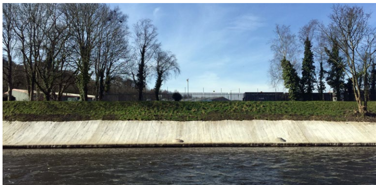
Figure 4.5 CC deployed for bank protection
