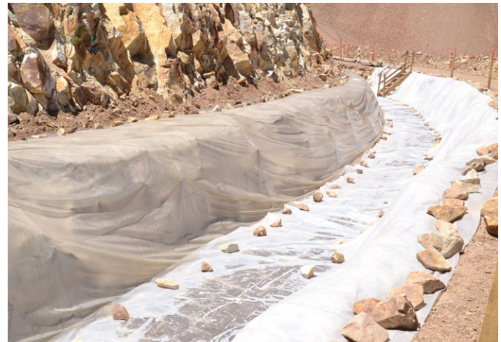
Figure 9.1 Plastic sheeting on CC during curing
