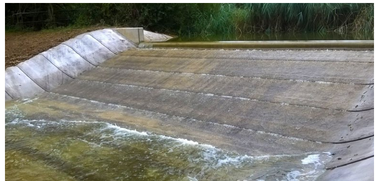
Figure 4.6 CC deployed for a spillway
