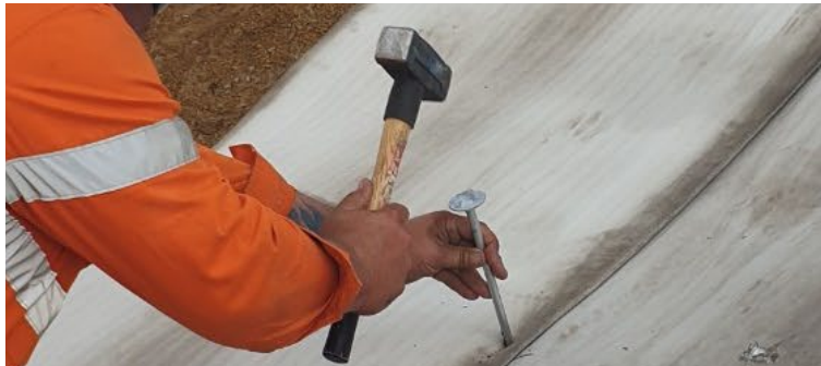
Figure 7.3 Round head peg intermediate fixing
