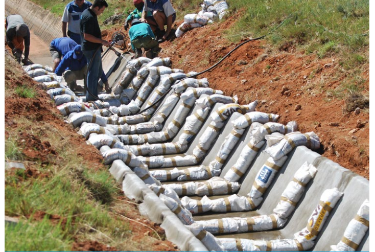
Figure 8.4 Sandbags to compress joints at setting
