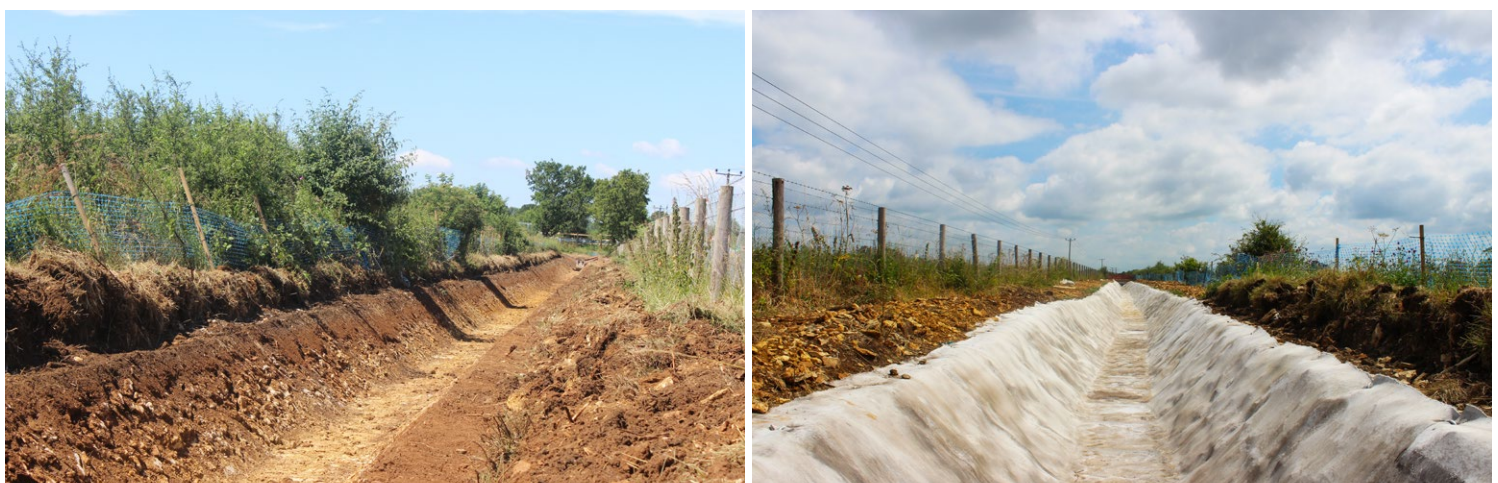
Figure 3.2 CC channel prepared with a ditching bucket (images taken before and after install)
