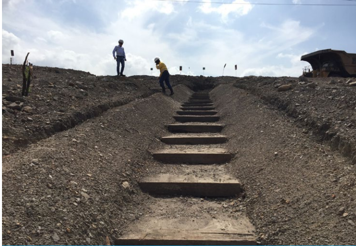
Figure 8.3 Form baffles by laying CC over structures
