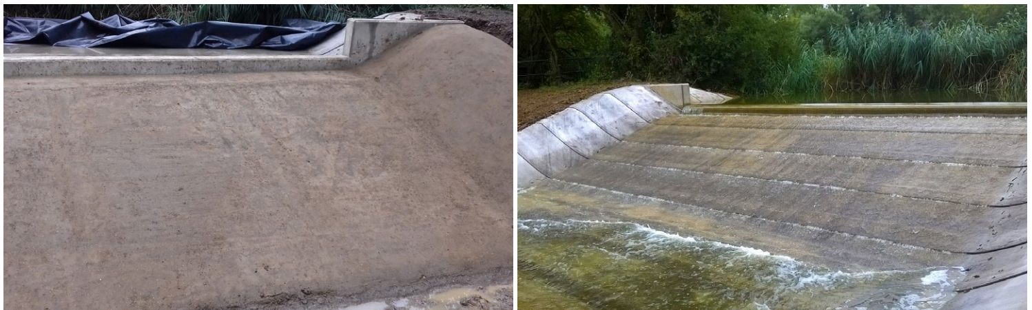
Figure 3.1 CC spillway installed on a trowelled sharp sand substrate (images taken before and after install)
