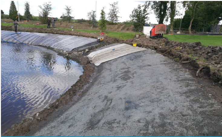
Figure 3.3 CC bank protection on a raked soil substrate (images taken before and after install)
