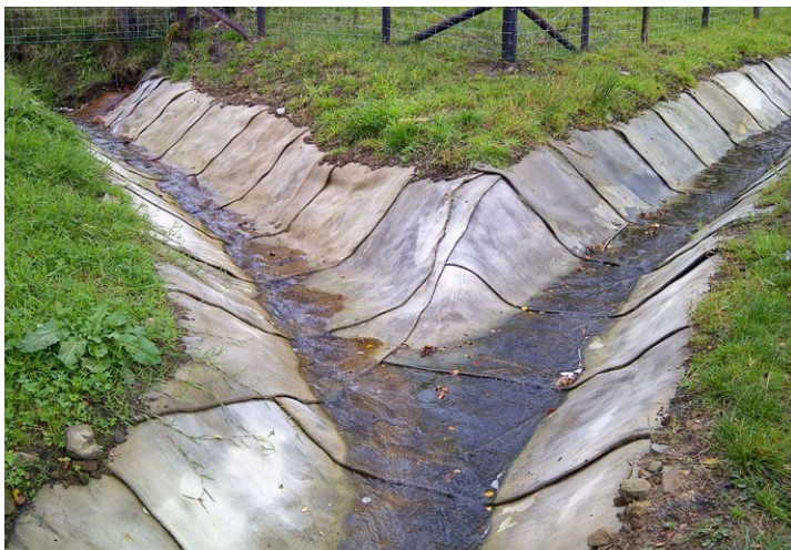
Figure 8.7 CC manipulated to form junctions
