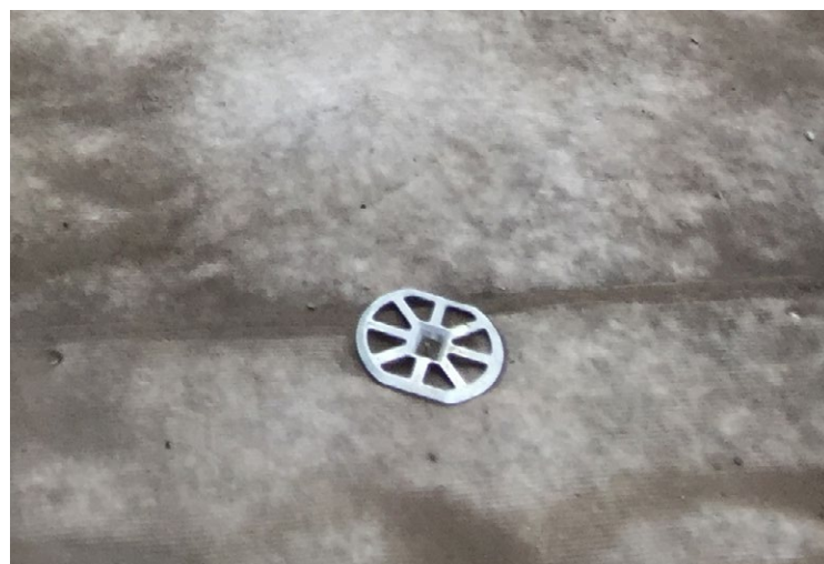
Figure 7.2 Earth percussion anchor intermediate fixing
