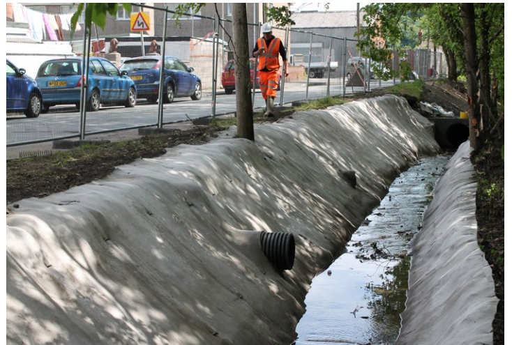
Figure 8.6 Retrospective pipe penetration
