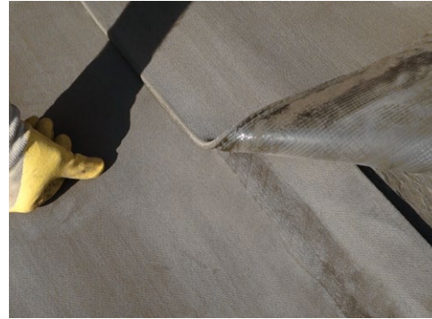
B. Too fast / Too cold: Joint will pull apart after cooling without causing delamination of the PVC.
